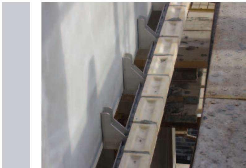
Relieving angle fitted directly to PFSolutions wall
