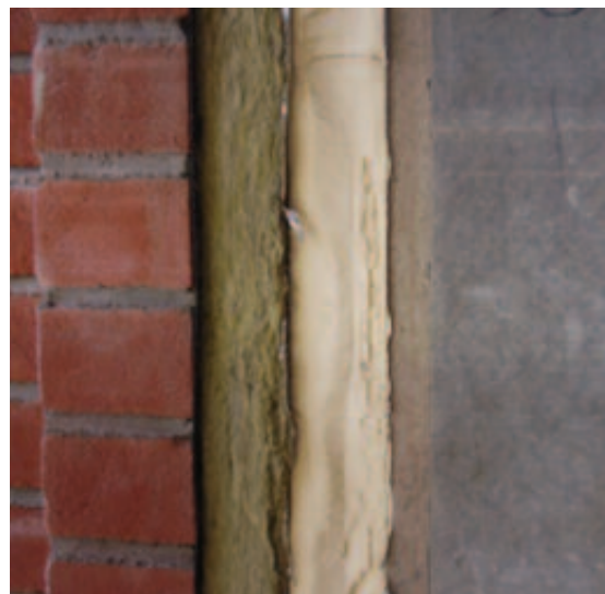
Typical external wall with closed cavity detail
